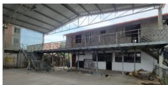
Mezzanine Under Construction
